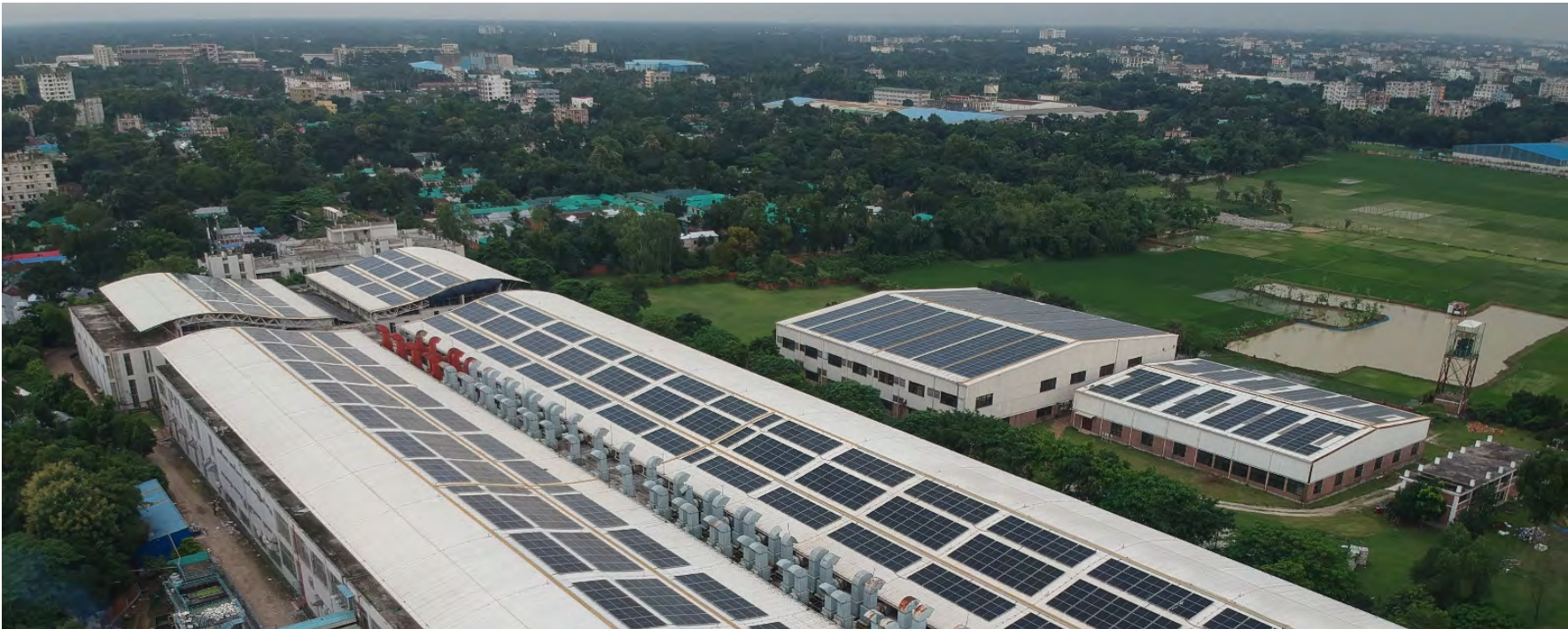
Solar panels in Bangladesh at one of our factory partners.
