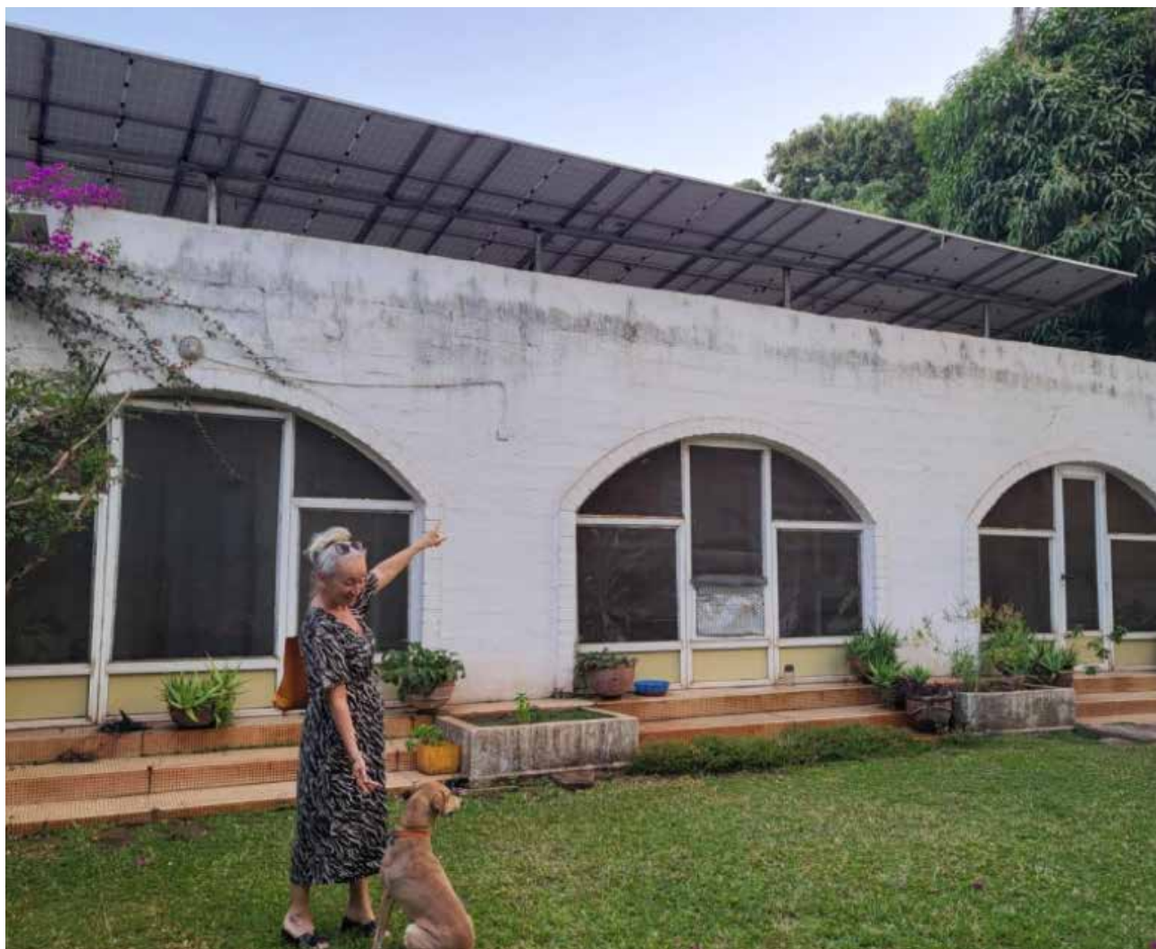
Solar installation powering the Country Director's residence in Bamako, Mali. Photo: Norwegian Church Aid
