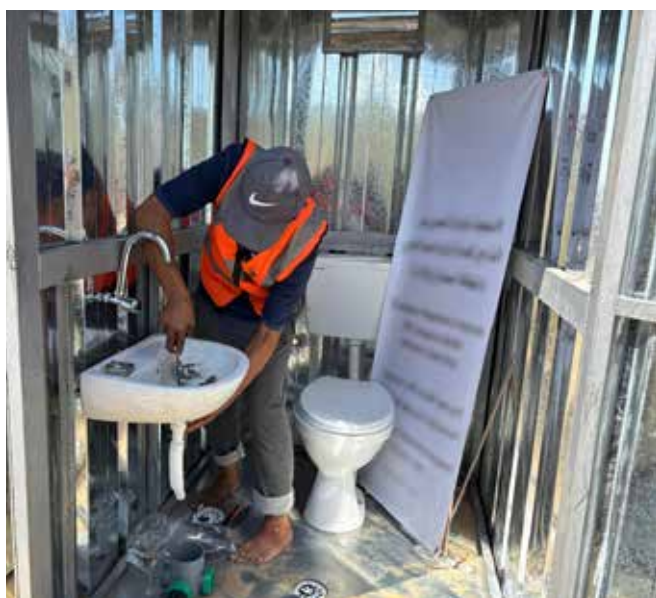
Construction of accessible sanitation facilities for persons with disabilities in Gaza. Photo: Norwegian Church Aid, Palestine
